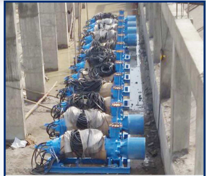
• SubCF pump sets installed in Suction Trench even as the Civil works are ongoing.
