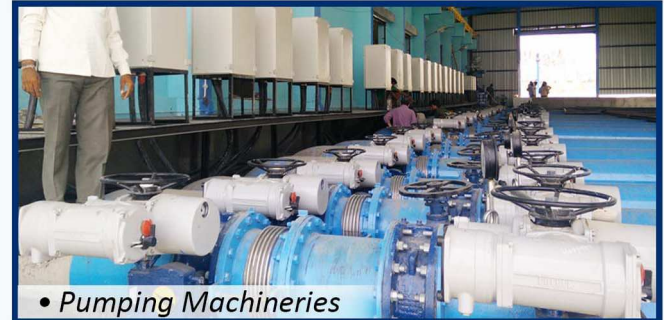
• SubCF pump sets installed in Suction Trench even as the Civil works are ongoing.
